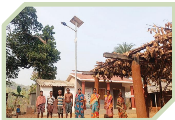
Installation of Street Light at Kaladu
